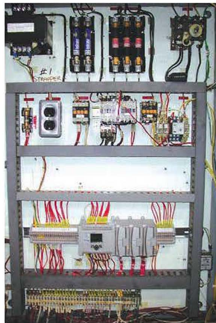
The panel above is a compressor control system retrofit for a plastics manufacturer. The panel to the left is a system upgrade for a pallet strapping operation.
