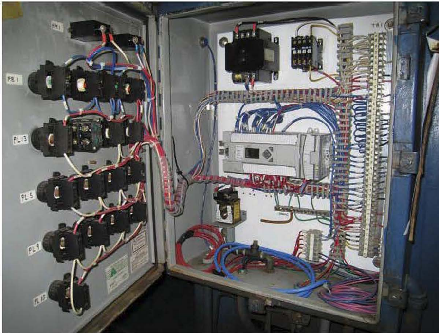
The panel above is a compressor control system retrofit for a plastics manufacturer. The panel to the left is a system upgrade for a pallet strapping operation.
